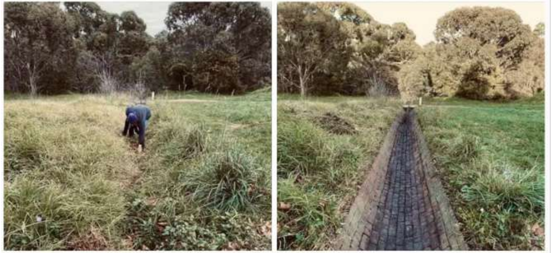
Source 3. Before and after the clearing of the Victorian swale drain below the old Asylum (now a gated community).
