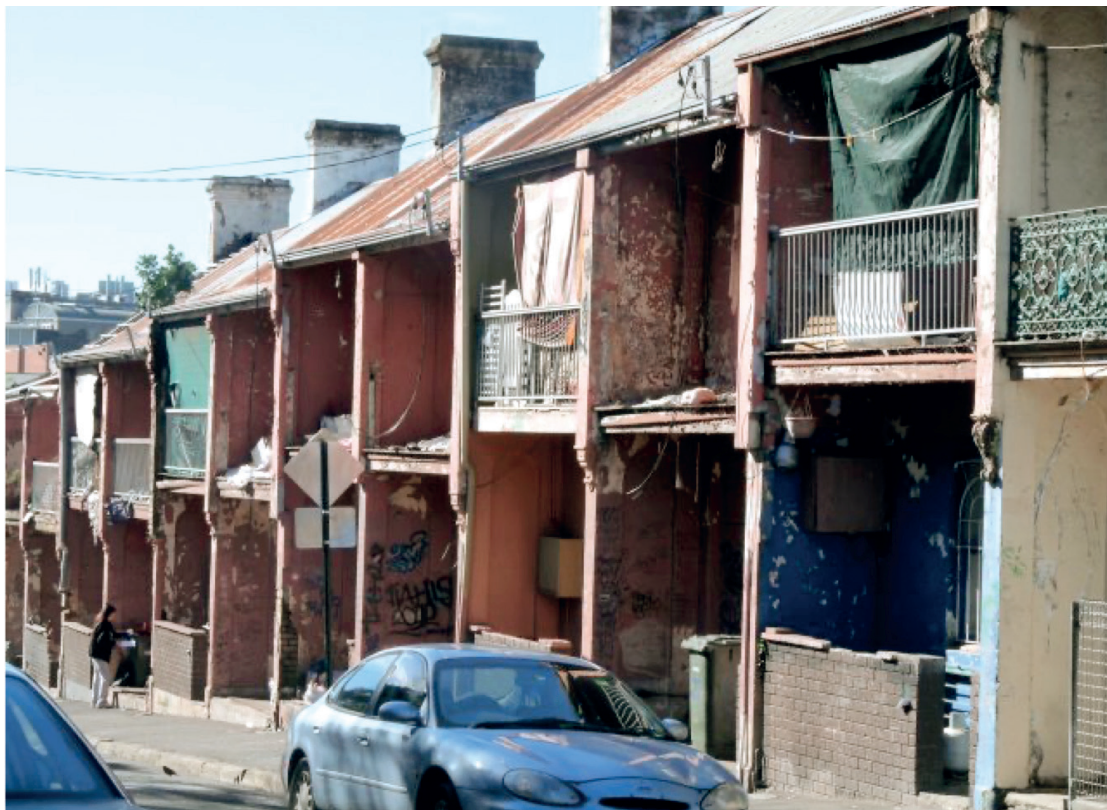
Figure 4: Eveleigh Street before demolition. The last tenant departed the Block in 2004. By 2019, the entire site had been cleared.
