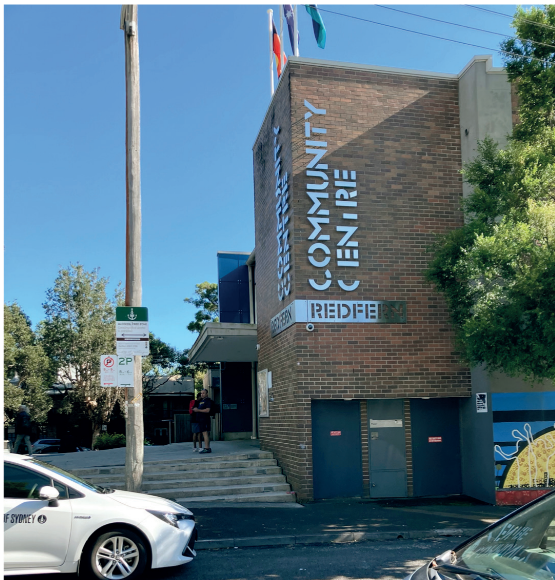
Figure 3: Part of the Pemulwuy Project, the Redfern Community Centre is a centre for Aboriginal social and cultural activities, surrounded by a landscaped park with an amphitheatre and a children's playground. It was formerly a printing factory, next to a disused timber yard and corner shop dating back to 1881. The opening of the Centre in 2004 occurred during a transformative period on the Block.
