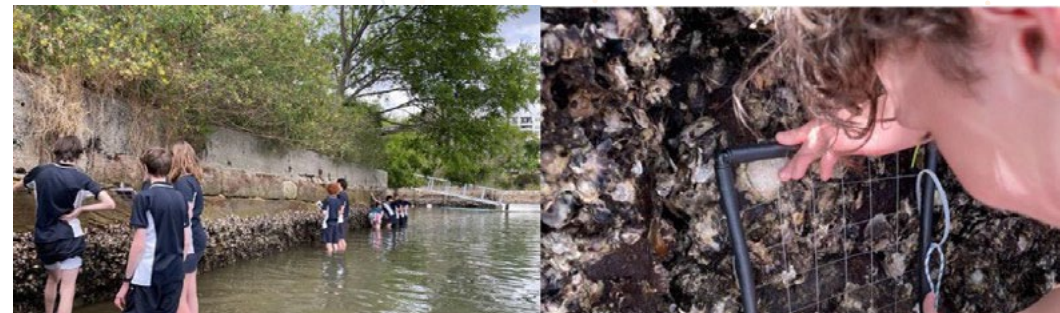
The existing seawall (above), and student participating in the pre-installation surveys
