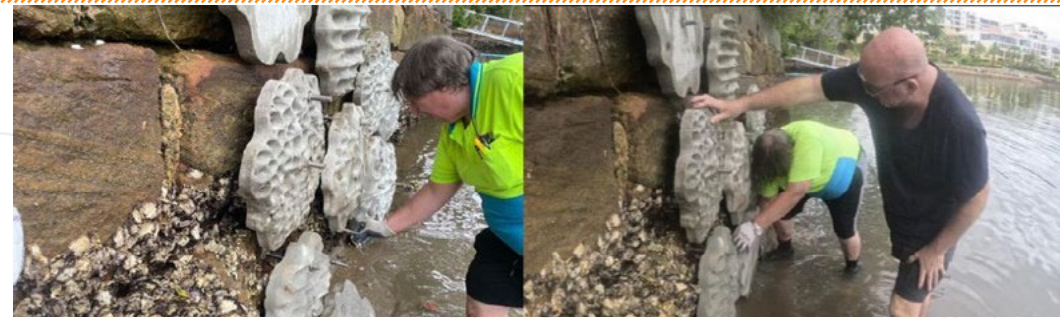
Installation of the Living Seawall panels
